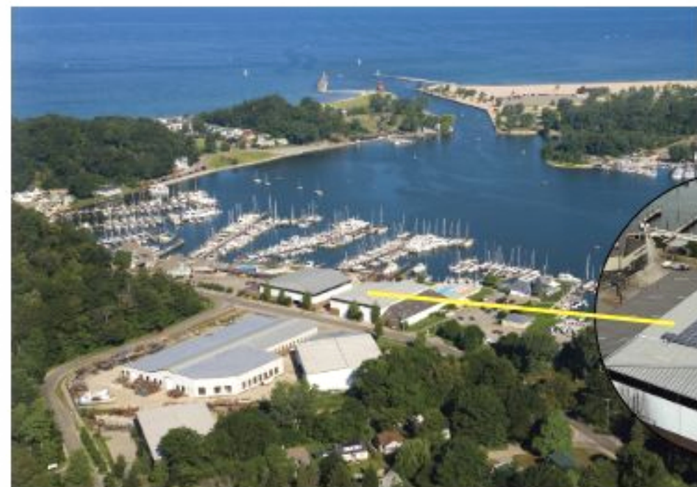
Boat storage buildings are ideal sites for solar panels. Below (clockwise) Wade and Kris Eldean; COVID aware celebrations on 4 th July; The new building with fire pit during the winter.
